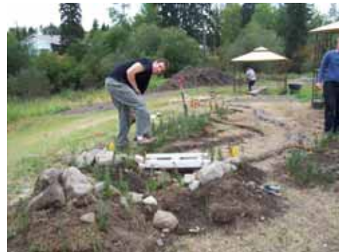
Working hard in the construction stages
